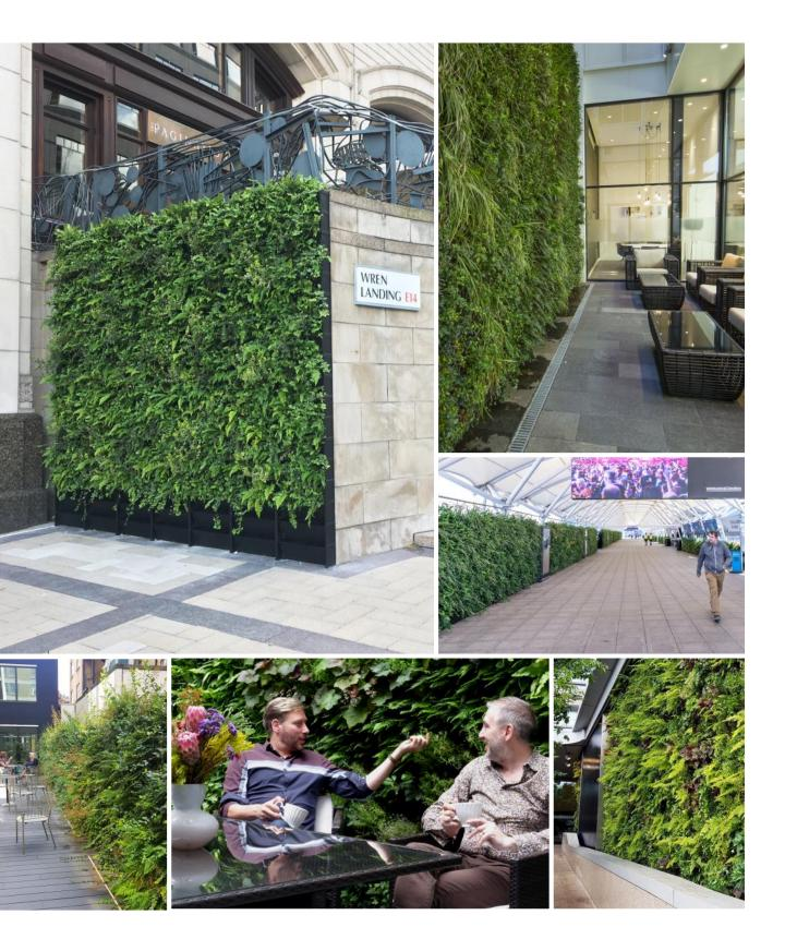
PlantBox **is** a cleverly simple living wall system designed with ease of installation, planting, watering and after-care in mind. The stackable trough assembly allows for small or large vertical spaces to be greened, with only the need to restrain the boxes back to a suitable wall or structure at height, and the integrated irrigation makes watering really easy.
