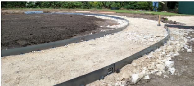
All of our edgings except our weathered steel (Cor-Ten effect) have a 20-micron Galvanised Zinc coating. Our (RAL) coloured edgings have a further 110-micron UV resistant polyester powder coating preventing colour fade, forming a durable scratch resistant barrier guaranteeing a 20yr plus product life.
