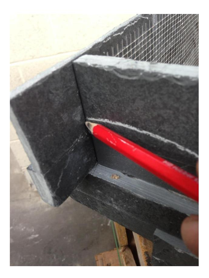
Where to cut on the rear of the panel; note the different pencil marks on the separate strips as each strip is cut separately.
