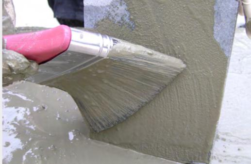
Failed paving is costly. The addition of a slurry primer to a paved construction is essential to guarantee a bond strength compliant with BS 7533.
