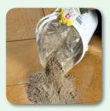
pour the mortar onto the wetted surface in small piles
