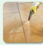
fully saturate the pavement surface
