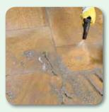
remove / clean any surplus mortar from the surface carefully using more water ...
